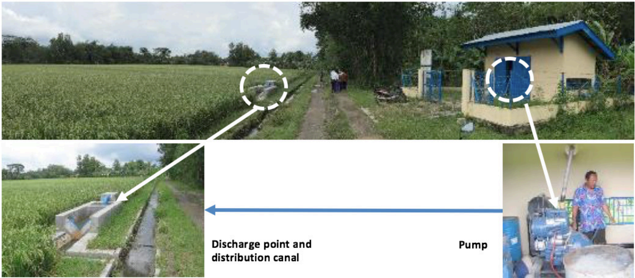
Figure 52. Groundwater bore wells for supplementary irrigation in rice field in Indonesia (GP-5.4i)
