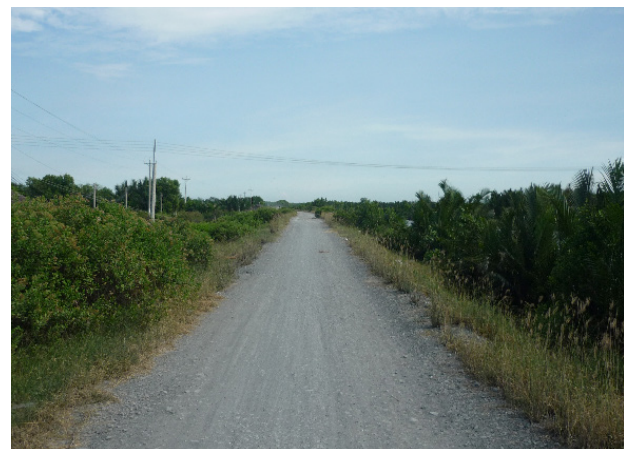
Figure 37. Polder dike including height for sea water level rise for protecting delta area of the Mekong River in Ben Tre Province, Viet Nam (GP-5.3c) Source: JICA Project Team
