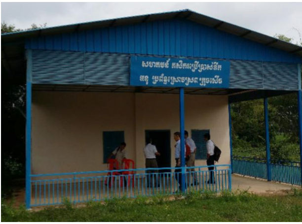
Figure 45. Office of a water user association in Cambodia (GP-5.4b)
