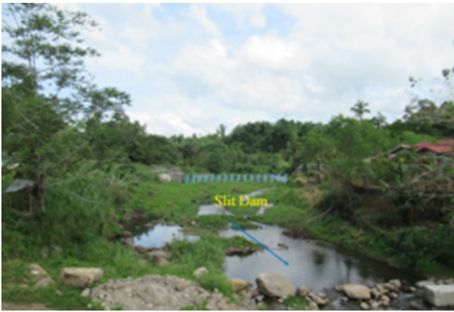
Slit Dam in the Anilao River Upstream Reach
