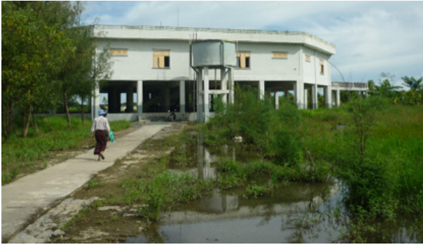
Figure 40. A cyclone shelter in Ayeyarwady Delta in Myanmar (GP-5.3f)
