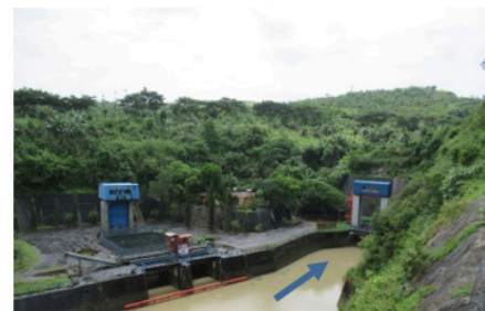
Phase I tunnel (Right) and intake of power station (Left)
