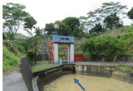
Phase II tunnel
