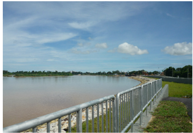
Figure 30. Pahang river in the downstream reach: River dike with river wall in the right bank side (GP-5.2b)
