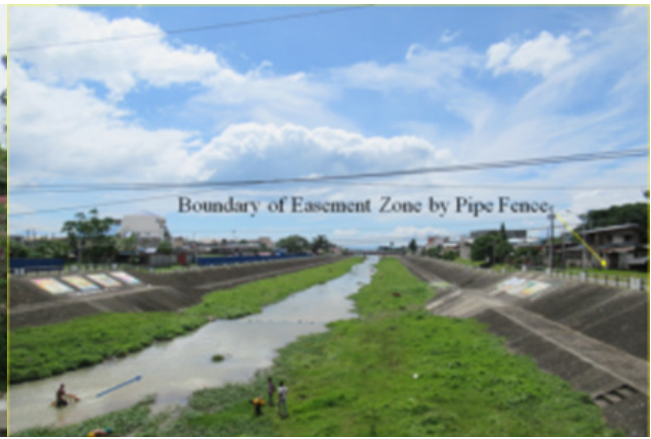
River Improvement in the Mid-stream to Downstream Reaches of the Anilao River
