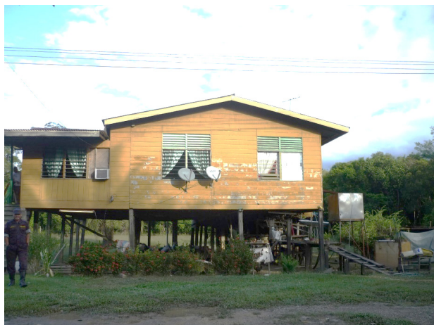
Figure 28. Elevated house beside the river (flood prone area with small flood velocity) (GP-5.1b)
