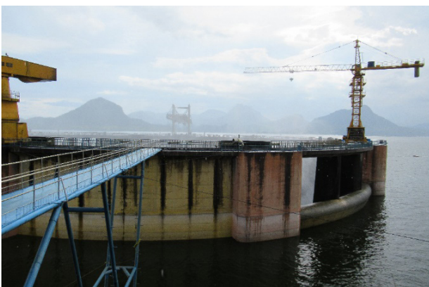
Figure 34. Jatilhur Dam (Reservoir and Spillway) in Citarum River, Indonesia (GP-5.2f) Source: JICA Project Team
